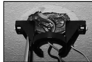
(3) Remove the stopper screw and loosen the set screws on the fan collar. Set the stopper screw aside for step (5).
